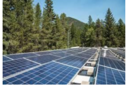
FIGURE . BALLASTED SOLAR PV ARRAY
