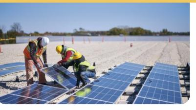
Ground mounted panels were utlized, due to their ability to be mounted at greater tilt angles than rooftop systems, which allows for better snow shedding and increased energy production in the winter months.
