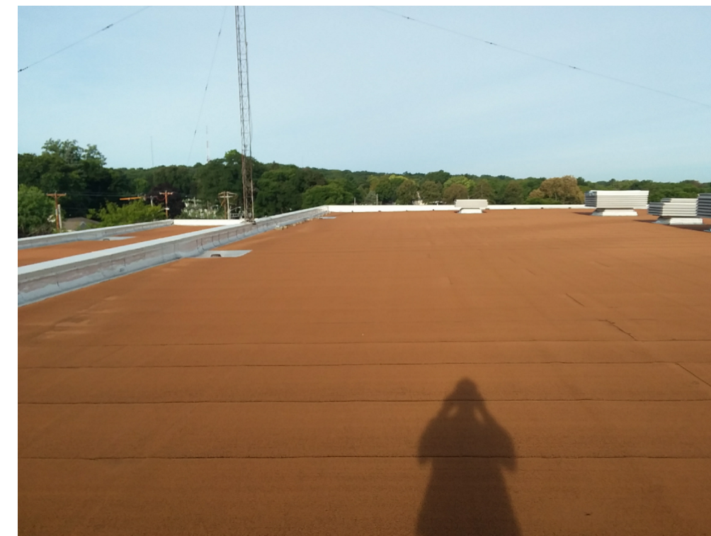
3 ROOF LOOKING SOUTHWEST NTS
