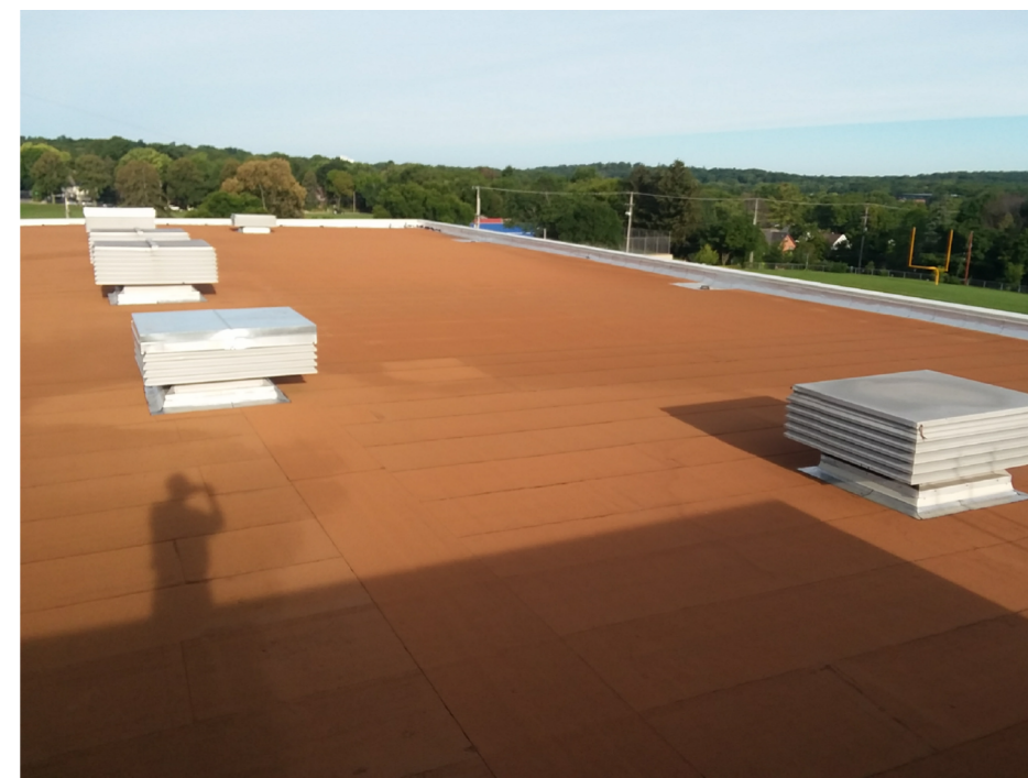
4 ROOF LOOKING NORTHWEST NTS
